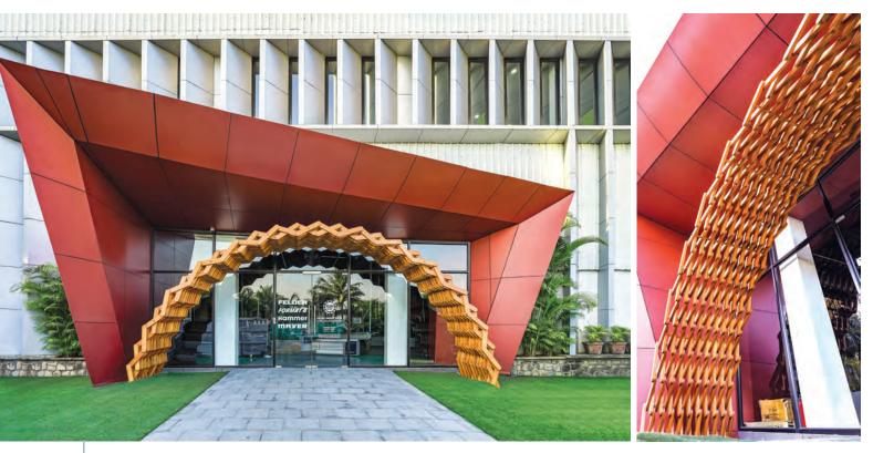
The geometry of the South-facing façade is broken with a coloured, slanting entrance portal (L) with vertical aluminium-clad fins to cut out excess light and heat. A 650-kg, 8-metre arch (R) made from Yellow cedar from British Columbia, Canada, was milled on Felder machines.
